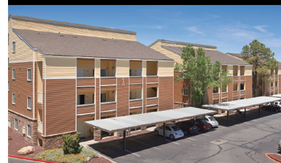
NEWLY RENOVATED EXTERIORS
