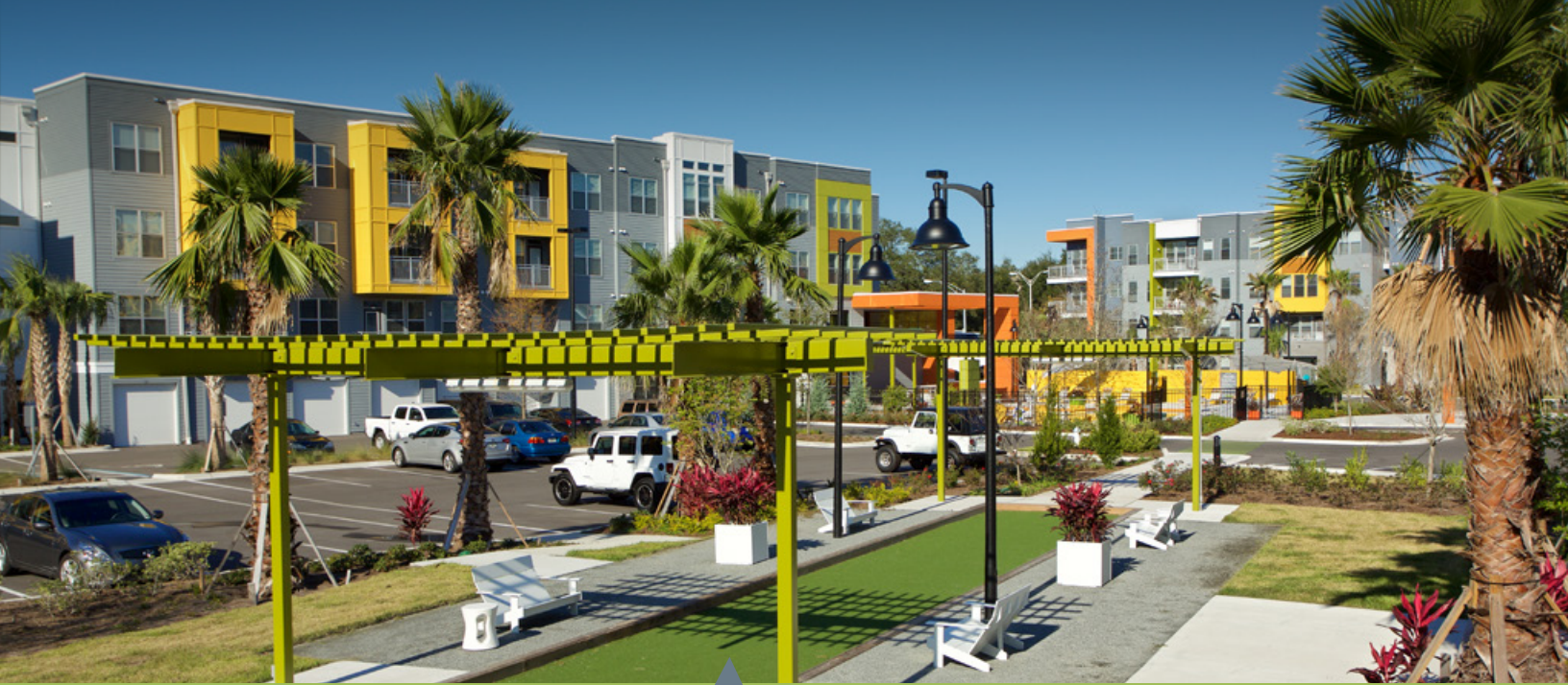
Modern Exterior Construction
