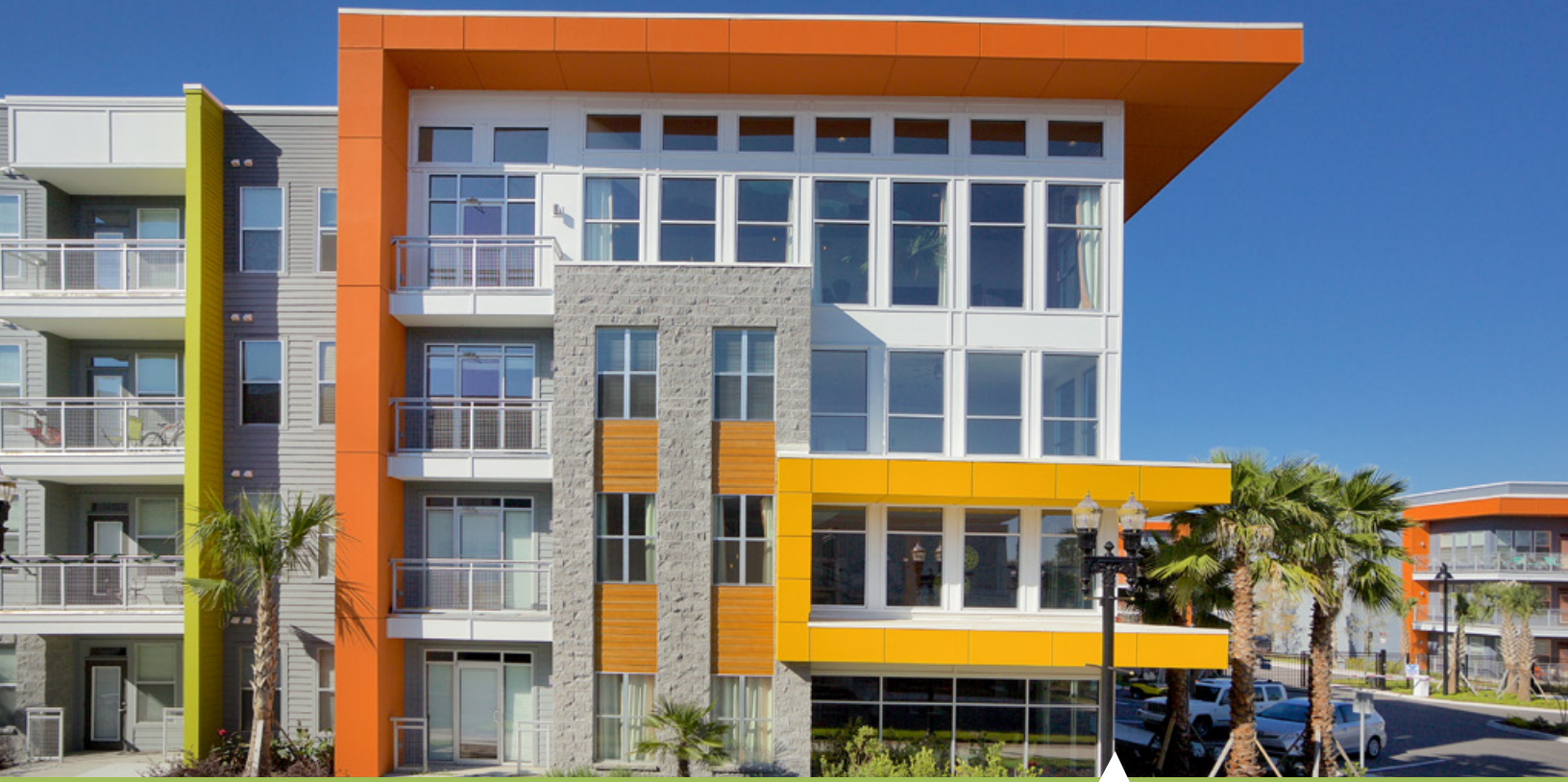
Modern Exterior Construction
